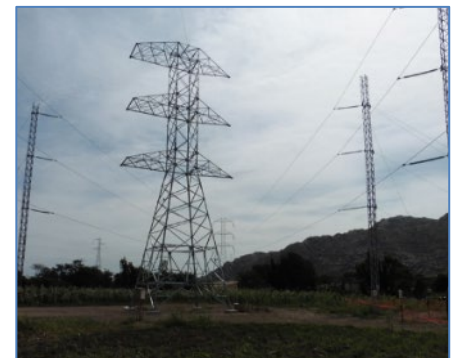
Montaje T14. Tramo Guadalupe – Reque
