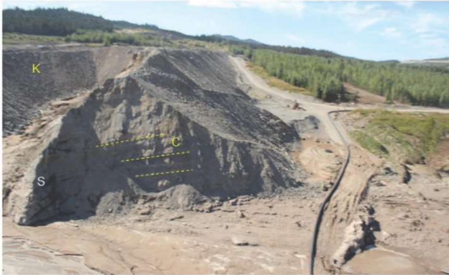
FIGURE 5.1.5: APPARENT BEDDING ROTATION ON LEFT ABUTMENT OF BREACH (SEPT. 4, 2014 PHOTO)
