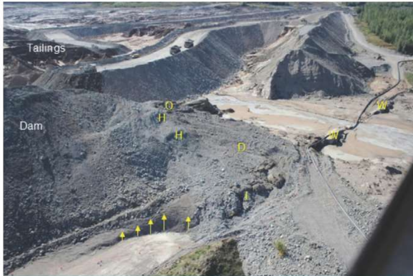
FIGURE 5.1.6: SLIDING-RELATED FEATURES AT RIGHT ABUTMENT (SEPT. 4, 2014 PHOTO)
