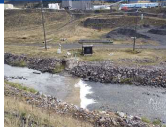
Flood Erosion Coal Mine BC
